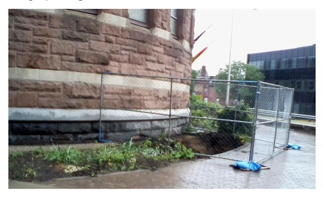
Test holes have been dug along the foundation of the church at the front (Maple Street) and side (parking lot), which to enable the contractors to assess the extent of the damage, done over time mainly by water seepage, to be repaired. The reconstruction will include replacing the plaza in front of the church and regrading and resurfacing the parking lot.
